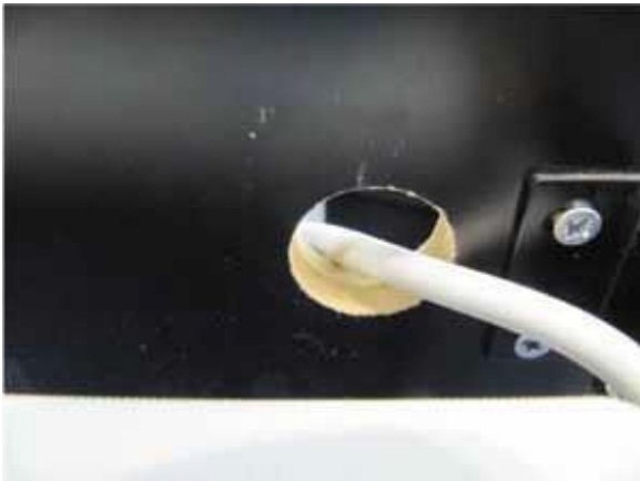
25mm hole for Somfy tail Installed with EMT 25 Grommet
