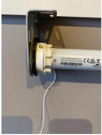
Step 3 - Alternatively, you may wish to turn the motor in the bracket from straight up and down to the next slot. Note: This will not stop the motor from working efficiently.
