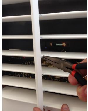
2. With a sharp blade, cut between the stile and the louvre that must be replaced carefully. Preferably do this on the hinged side of the door.
