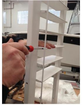
2. With a sharp blade, cut between the stile and the louvre that has to be replaced carefully. Preferably do this on the hinged side of the door.
