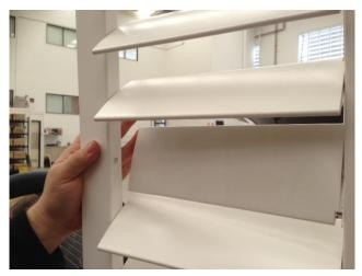
4. Place the spring-loaded pin from the louvre repair kit that would have been supplied with your louvre into the stile
