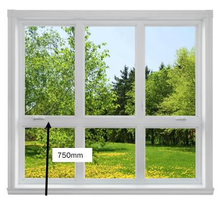
Example: Window Height is 2000mm with one Divider Rail required Divider Rail measurement is 750mm
