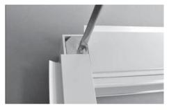
• Tighten the corner bracket screw.
